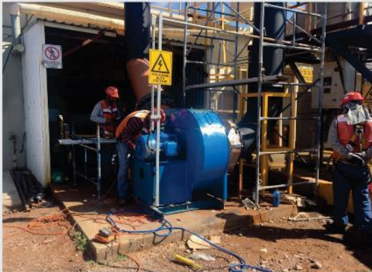
First Majestic – Santa Elena Scrubber gases repair, assay Laboratory
