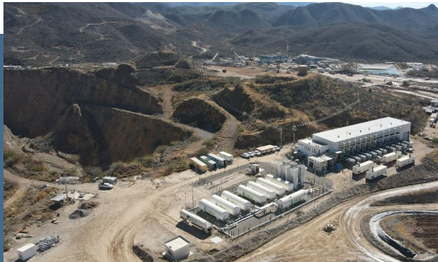
First Majestic Power generation (19.5 MW) plant and natural gas storage tanks
