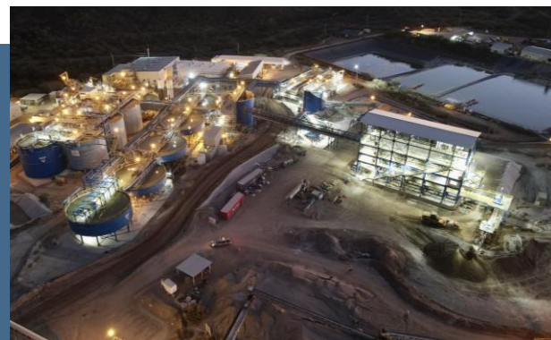
First Majestic Dual Circuit - Filter press OUTOTEC for 3200 tons of tailings per day of capacity, leaching tank and thickener tank
