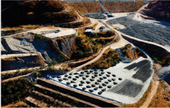
WHEATON RIVER MINERALS Remediation of Cupias tailings dam
